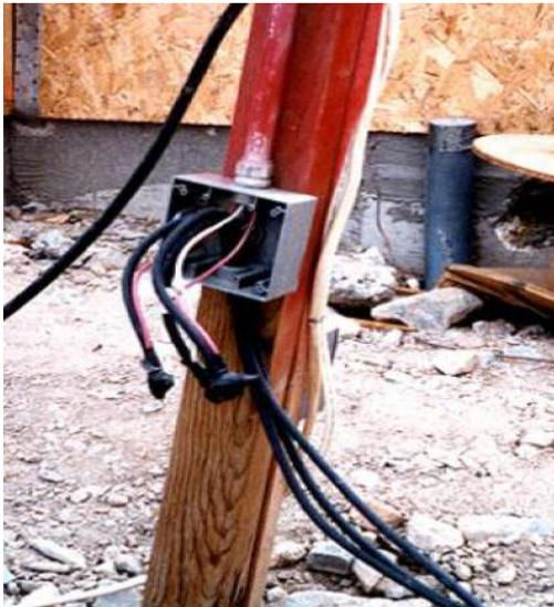
**Figure 11-2 Unsafe wiring installations**
