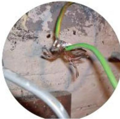
**Figure 11-3** Bad connections and exposed wiring
